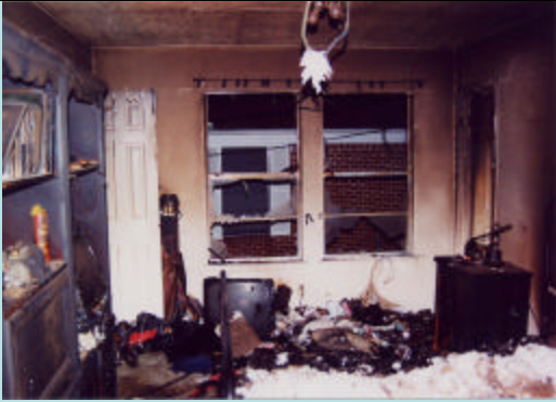
Fire room. Window vented from the outside with pike pole
