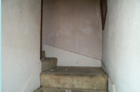
Looking up attack stairwell.
